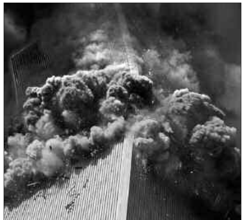
The explosions of the controlled demolition hurled materials from the cladding and the structure dozens of meters outwards.
